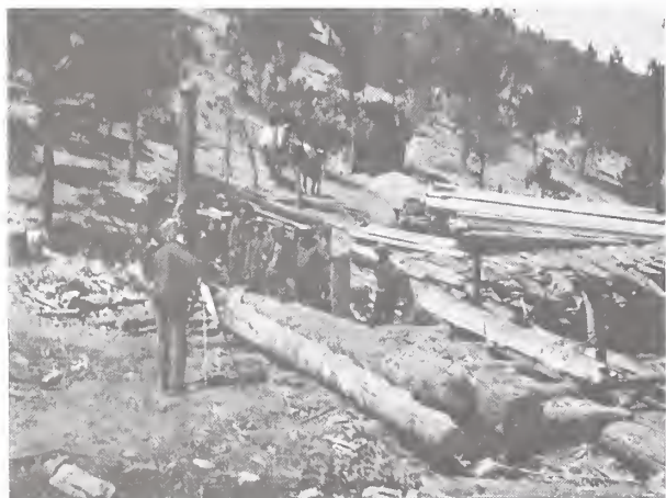
Figure 4. This steam-powered sawmill was used on the Reef around 1900. Note the beargrass-roofed shack in the background. Photo courtesy Arizona Historical Society (AHS #72762).
